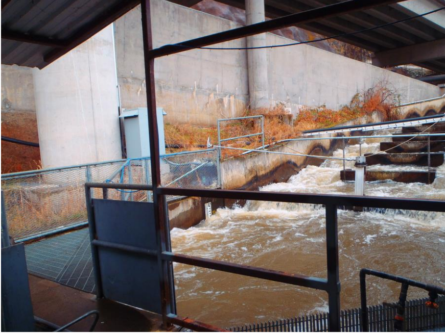
Photo 1. LWG fish ladder upstream picketed lead and weirs water level March 27.
